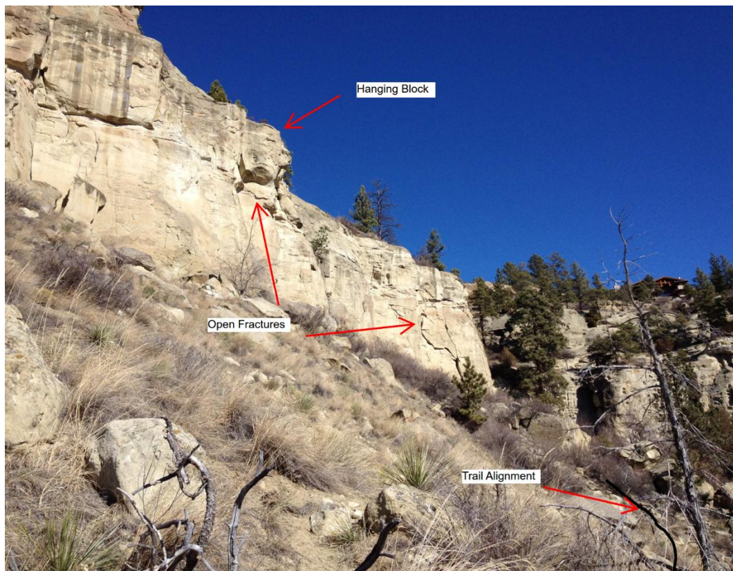
Looking north along cliff face above Sta. 25+00
