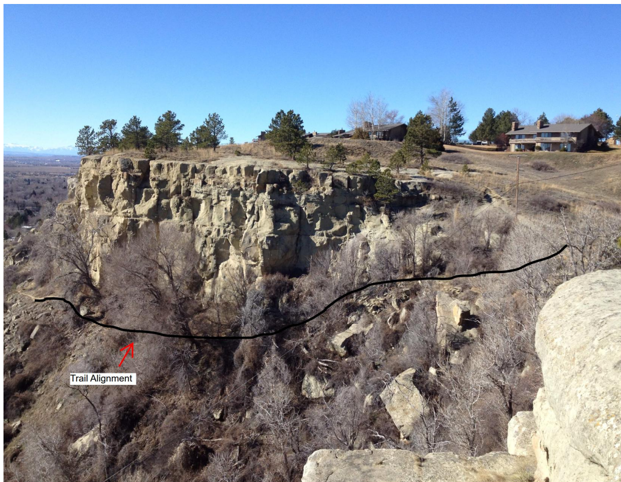
Upper portion of the Myers Trail alignment. Note the lack of large loose rock blocks that span the cliff face and the smaller cubical rock blocks at the top of the cliff that are actively failing.
