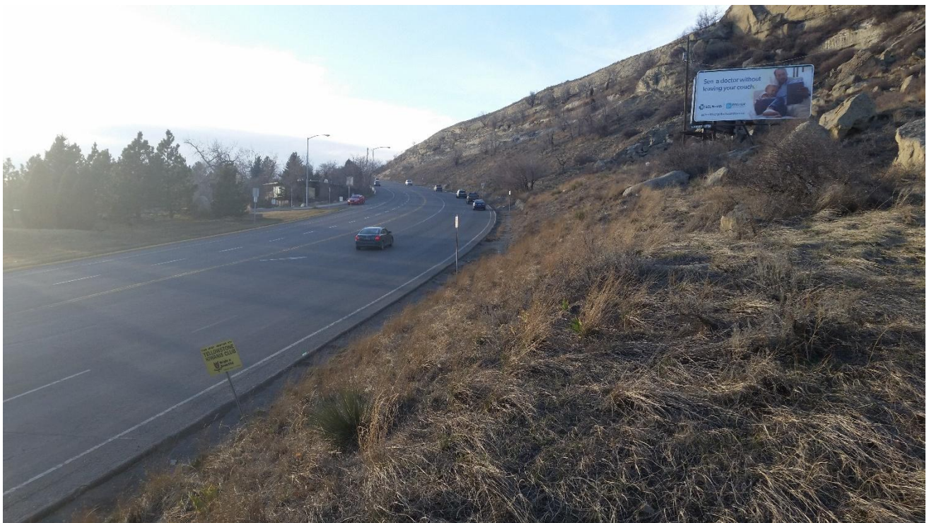
Looking west up North 27 th Street. Note, the stable nature of the rock slope. The trail alignment would be on the outside of the guard rail on the south side of the roadway.
