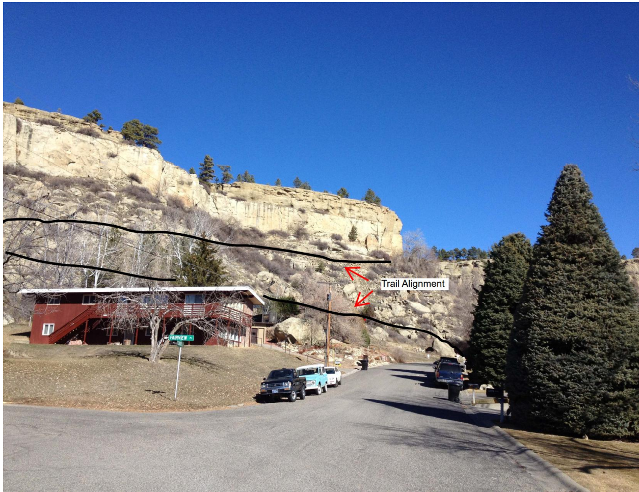
Cliff face above Country Club Circle. Note the relatively solid nature of the cliff face.
