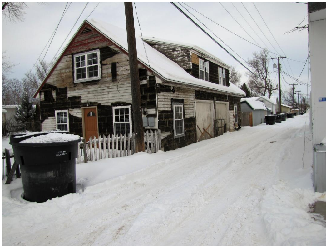
Looking East down the alley
