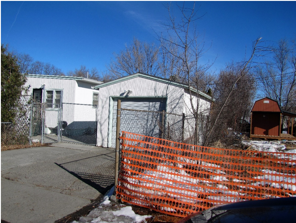
View northeast of subject property
