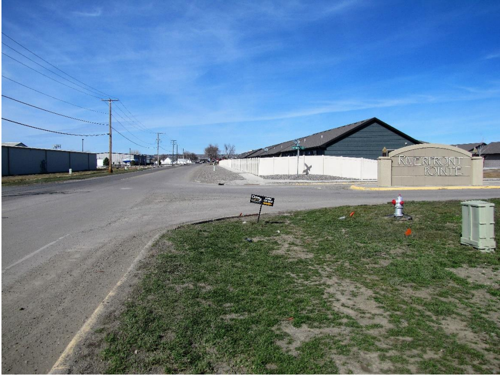
View north along Mullowney
