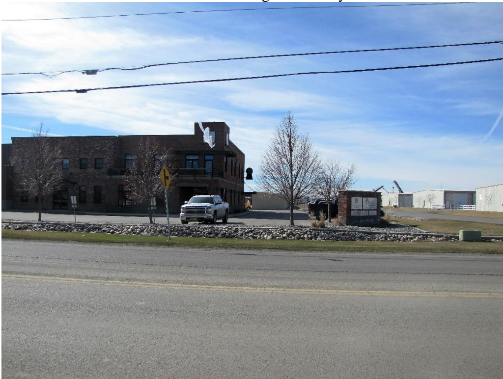
View west across Mullowney
