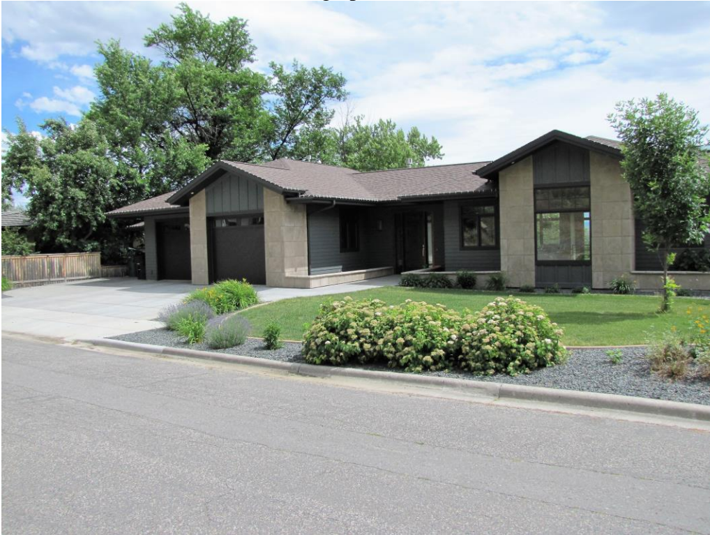
Looking south east
