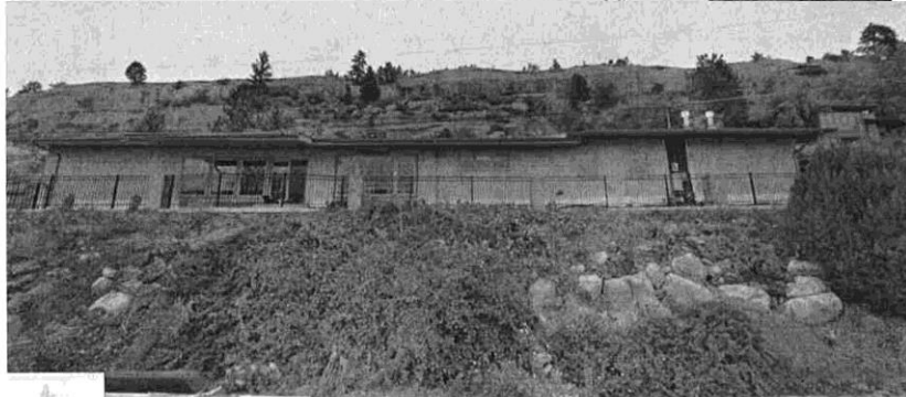
PHOTO 'B', 1425 Granite Ave. (adjacent property to west of subject property)
