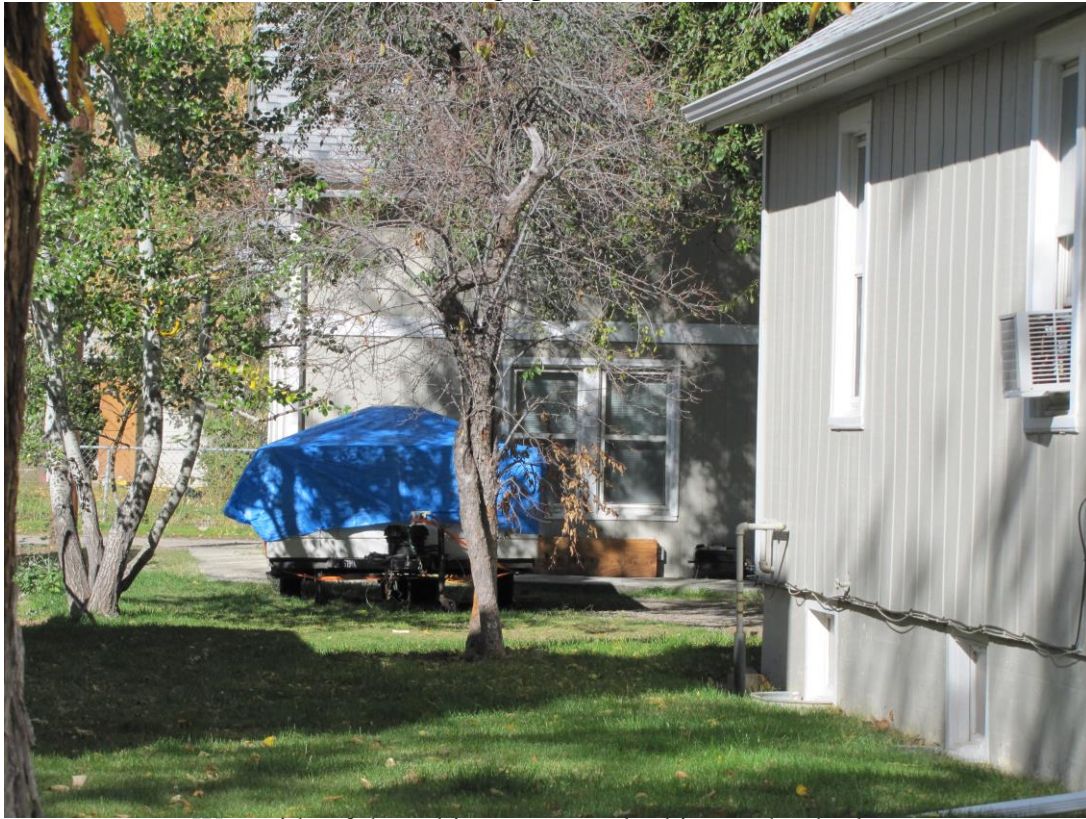
West side of the subject property looking at the duplex
