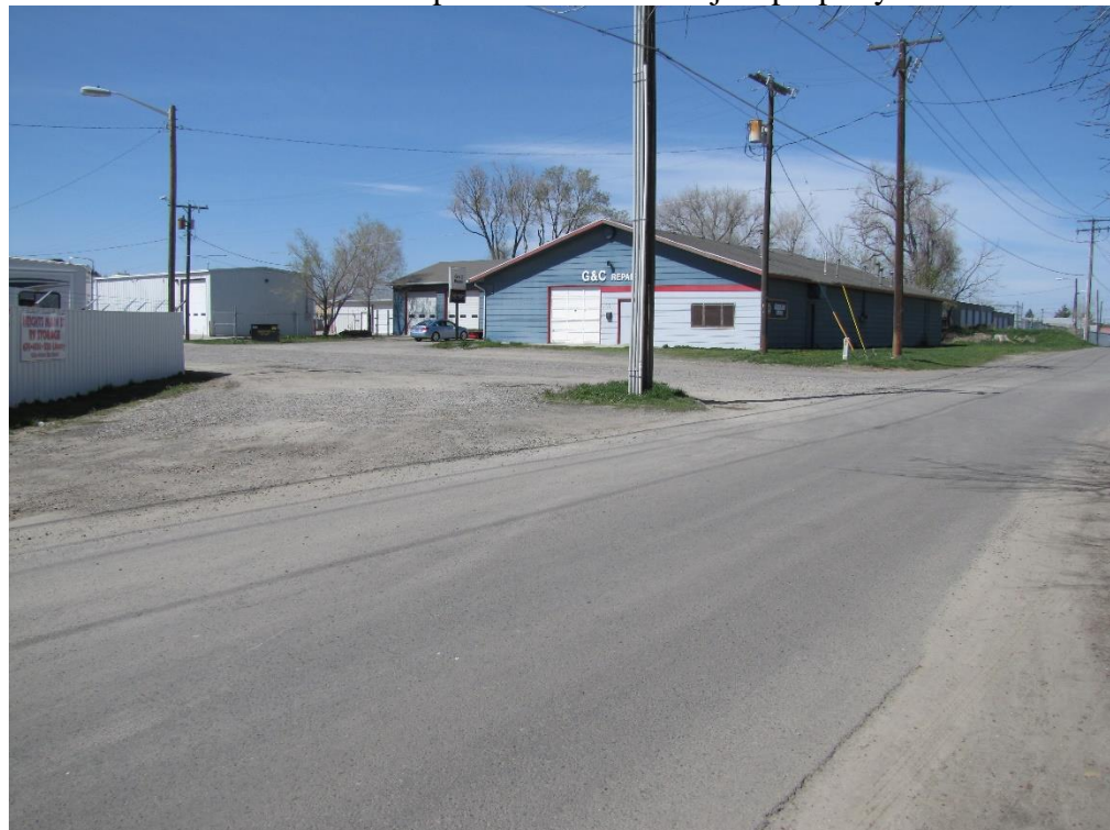
View north and west to auto services on west side of Lincoln Lane
