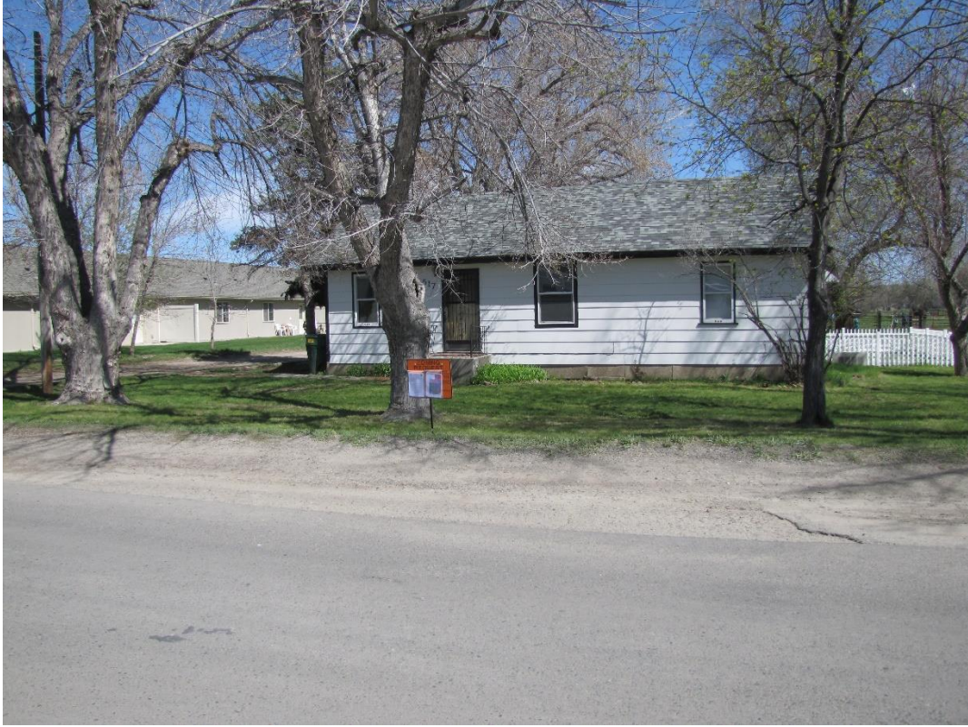
Subject Property – view from Lincoln Lane
