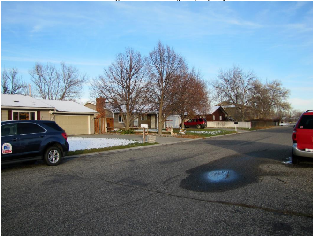
Looking north across Lynn Avenue
