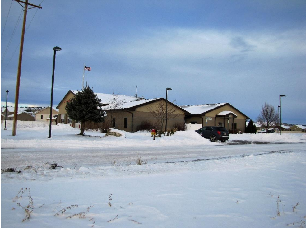
Fire Station #7 on 54 th St West
