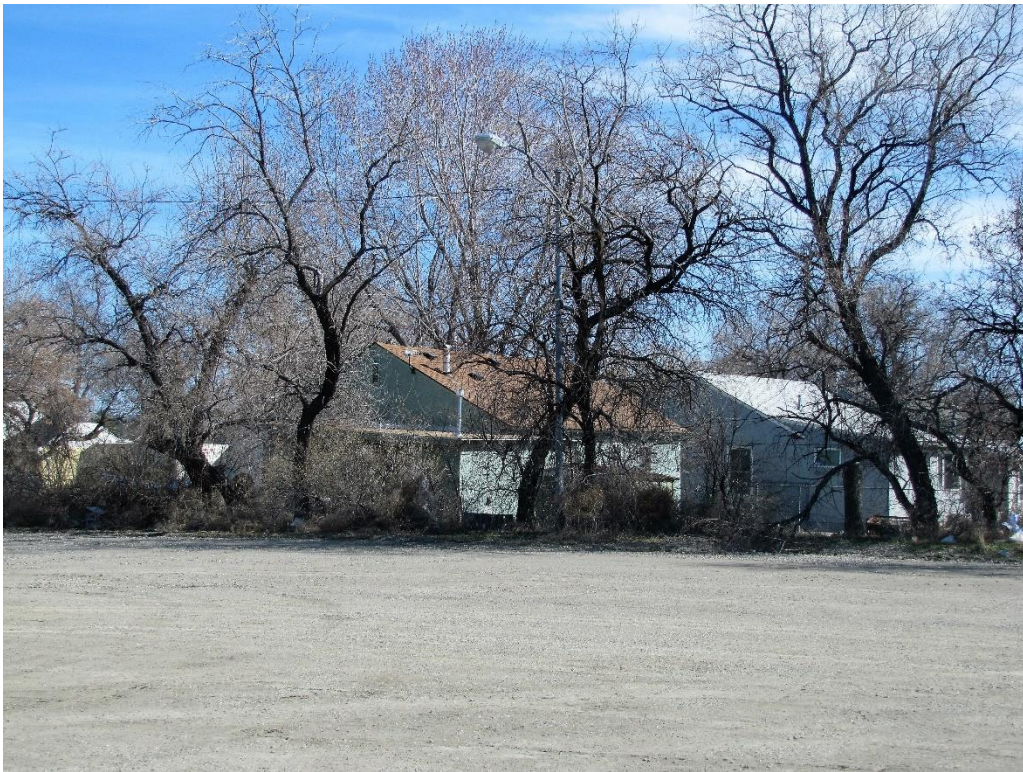
View south east across subject property from Laurel Road
