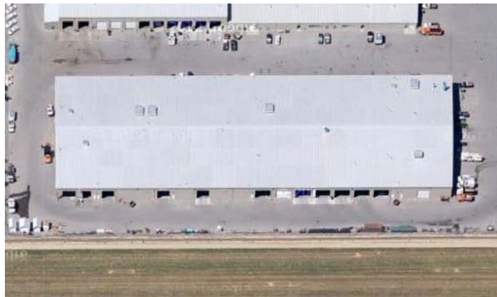
SOUTH SIDE OF GARAGE BUILDING AT BOC
