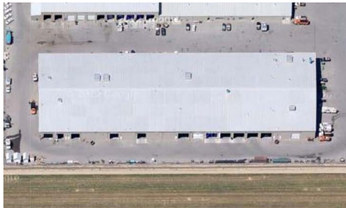
SOUTH SIDE OF GARAGE BUILDING AT BOC
