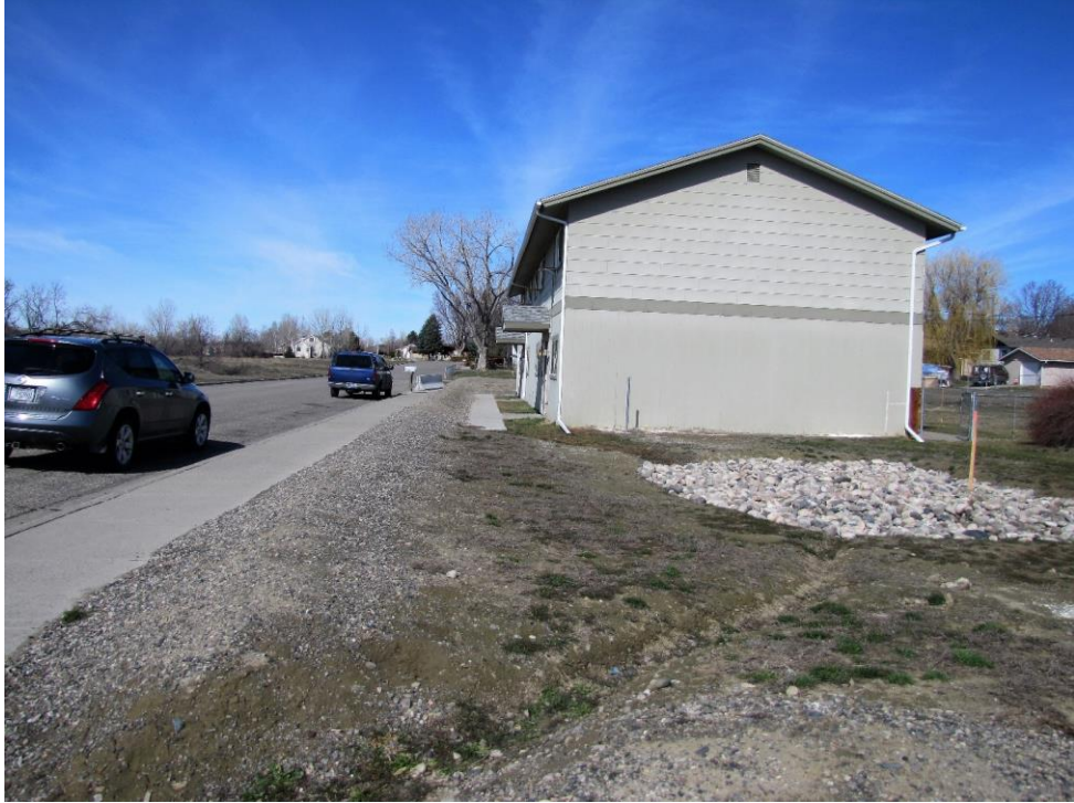
View from the corner of Cody Drive and Covert Lane looking north
