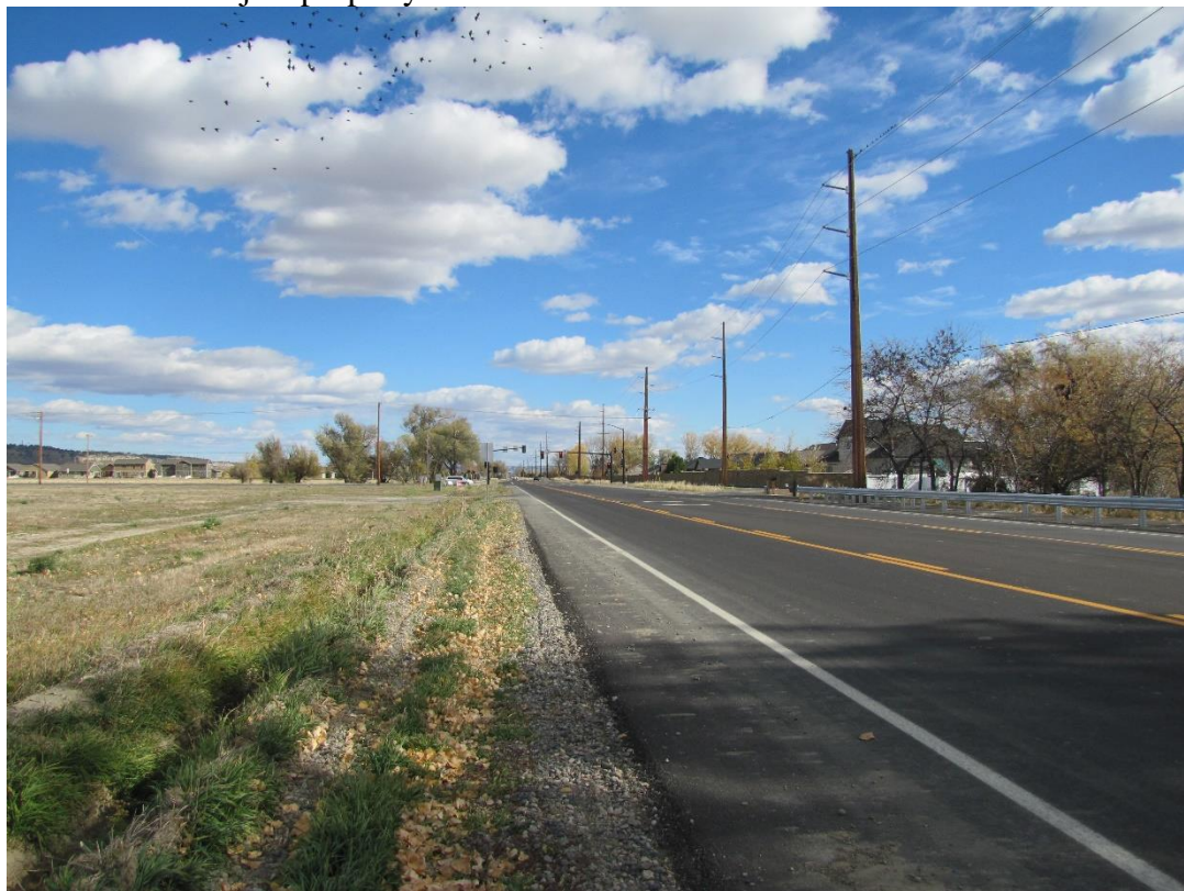
View east along Grand – new traffic signal
