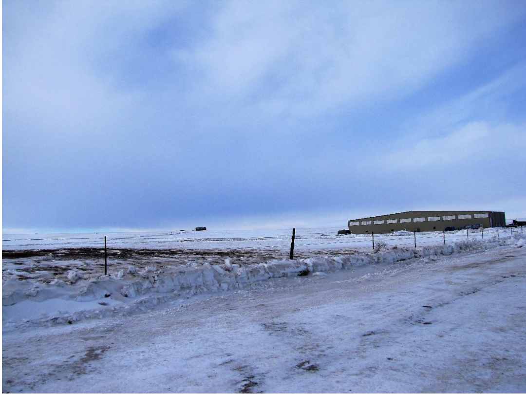
View of heliport from access road just north of landscape berm
