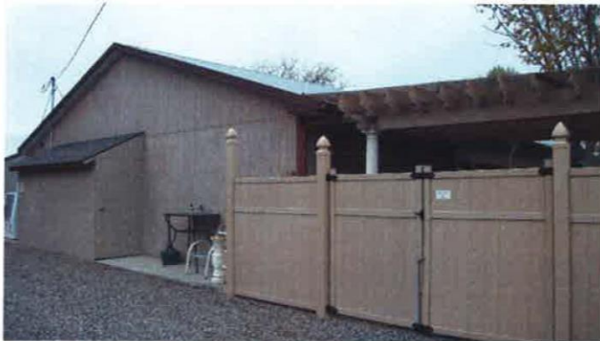
Pavilion Off Parking Area
