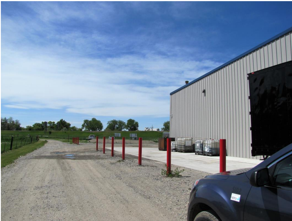
Looking west along Kimble Road Subject property to the left
