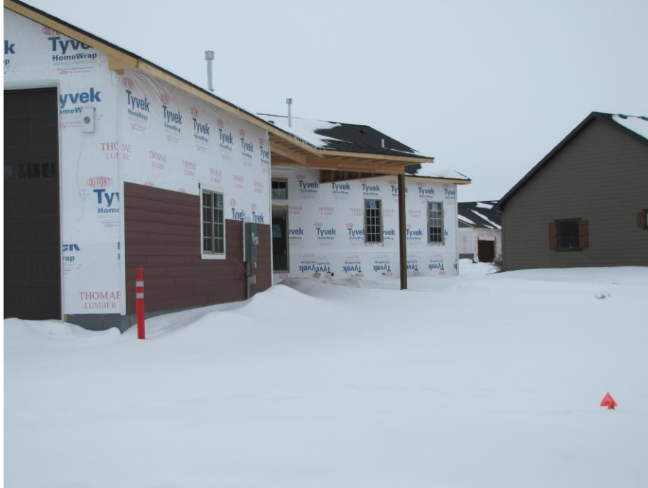
Covered patio, construction started
