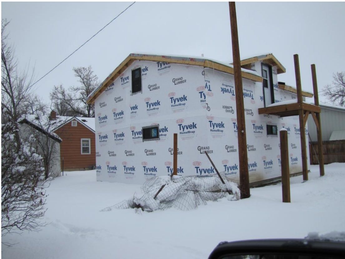
Looking from alley to new garage/art studio structure
