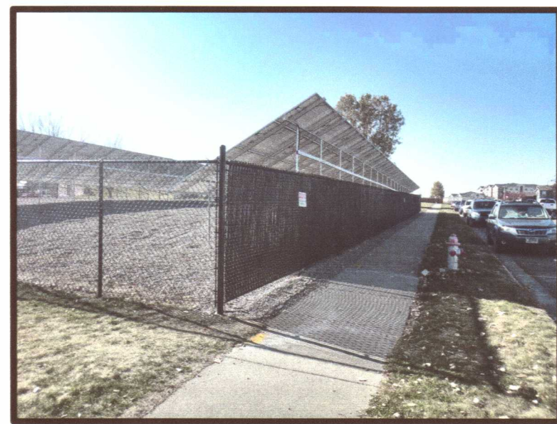
PHOTO 1: NORTHERN PHOTOVOLTAIC ARRAY, STANDING WITHIN ROW AT INTERSECTION OF SIESTA AVE AND DRIVEWAY, LOOKING WEST
