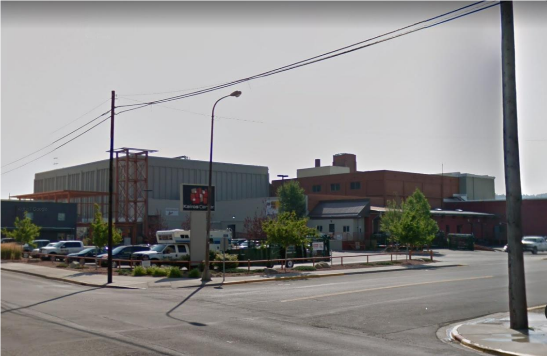
View east from 1 st Ave North at N 15 th Street
