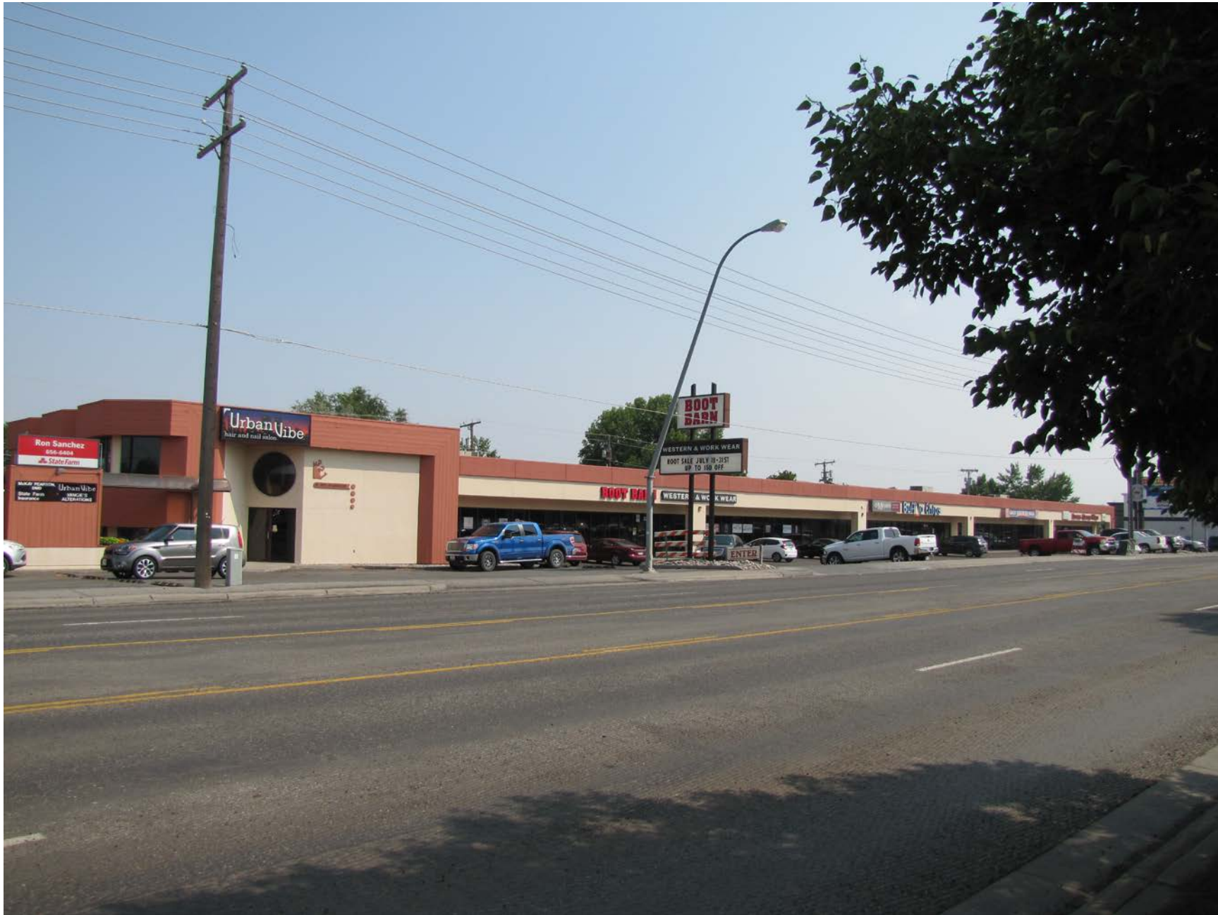
South east across 24th Street West
