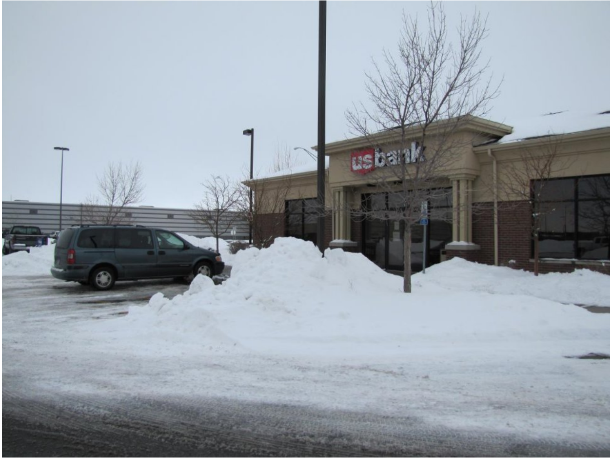
Neighboring property to the south
