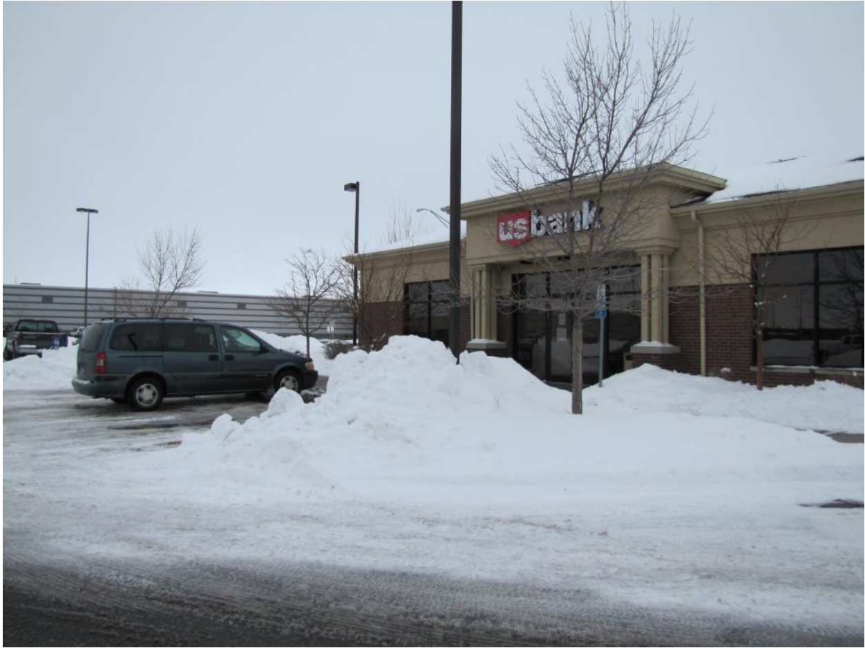
Neighboring property to the south
