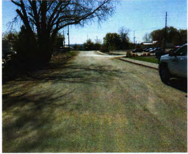
Commerce Way Facing East Toward South Billings Boulevard
