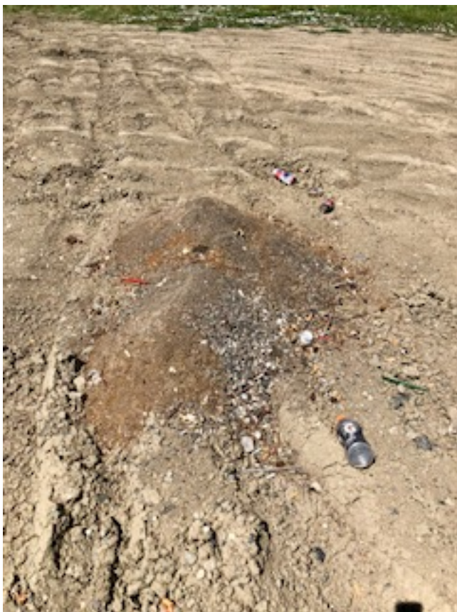
Small debris pile located on South edge of A35426
