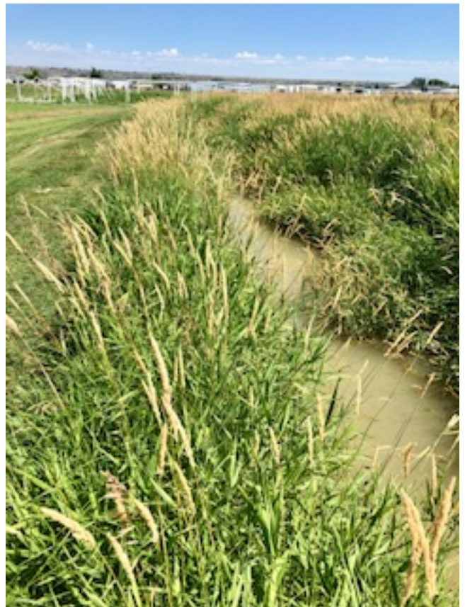
View of Suburban Ditch entering A35426 from South.
