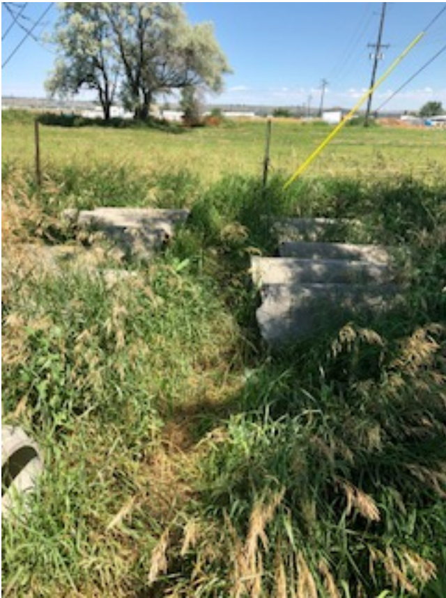
View of concrete pipe on North end of A35427
