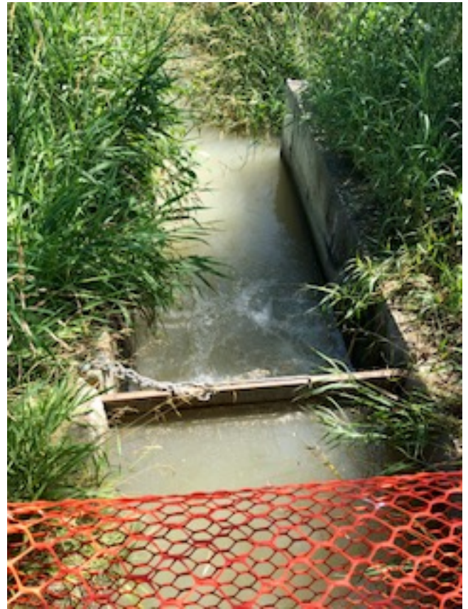
View of Suburban Ditch gate on COB land
