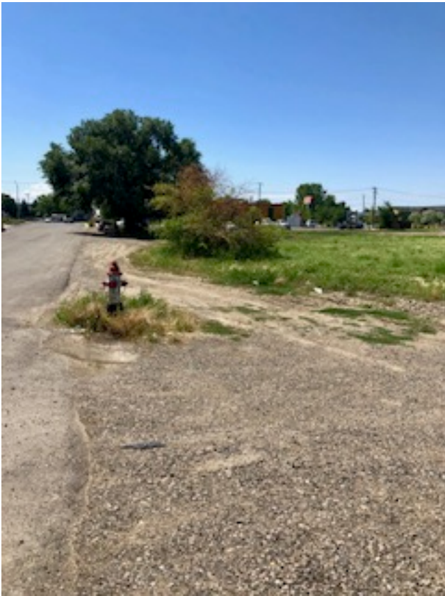
View from East side of A311390 looking South
