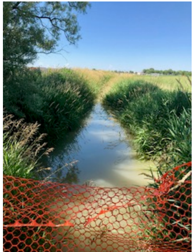
View of Suburban Ditch from Bridge looking West
