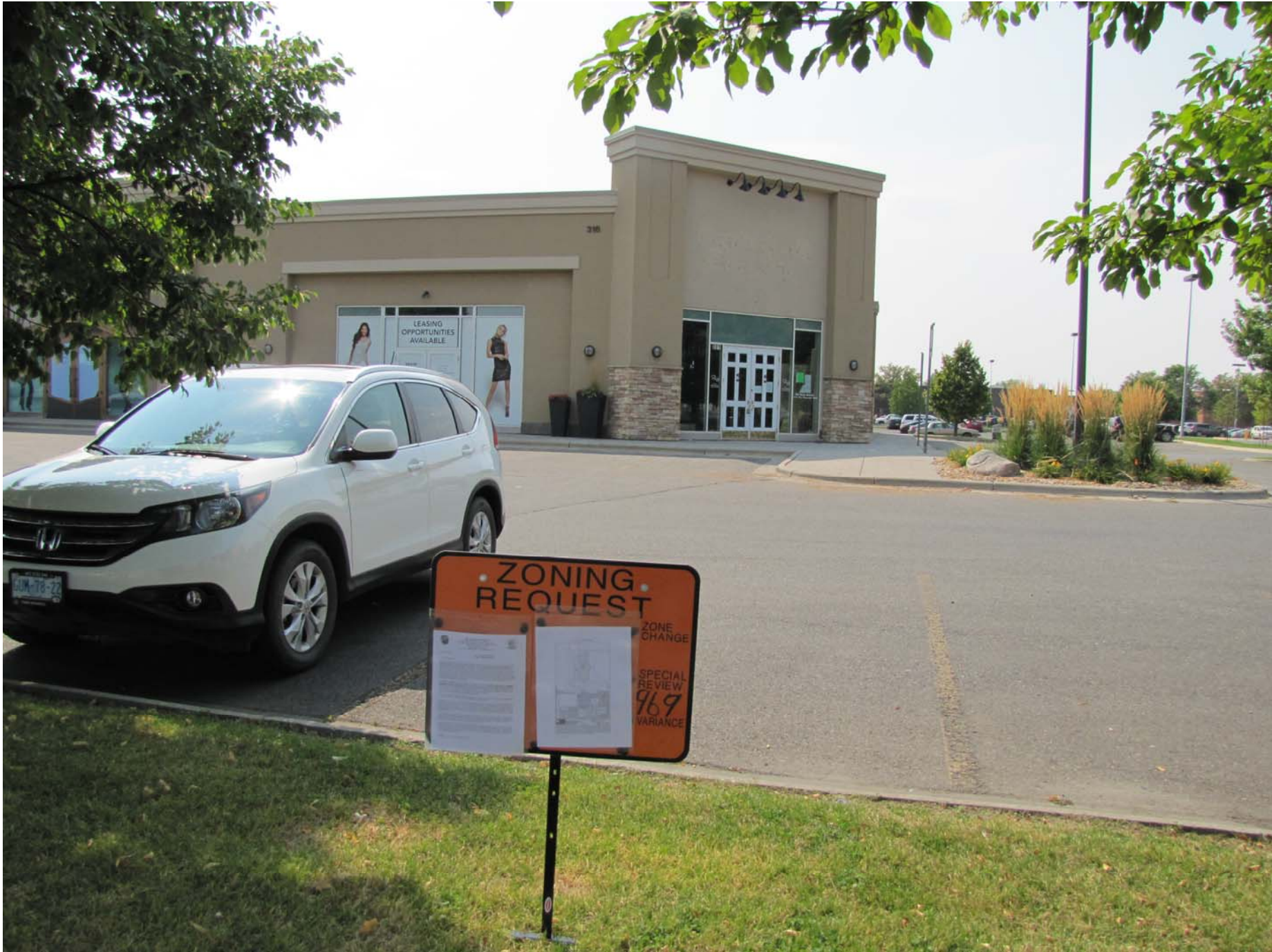
Looking west from 24th Street West
