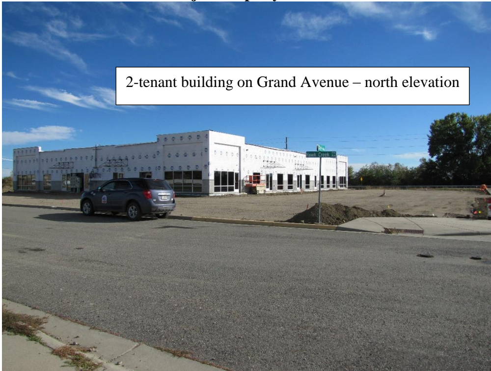
View south across Hawk Creek Avenue
