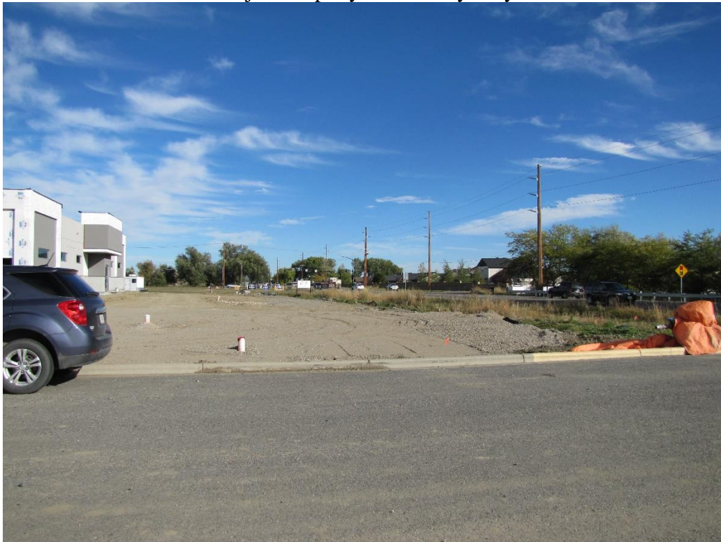
View east along front of new construction on Grand Avenue
