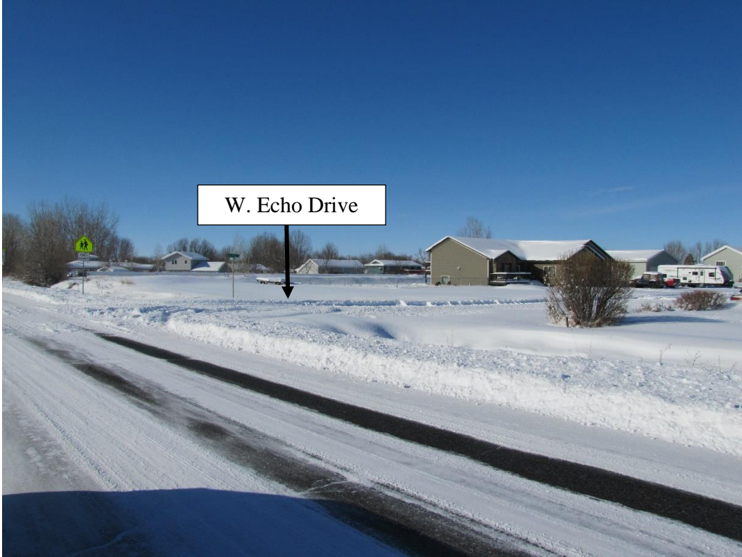
View west and north across Barrett Road
