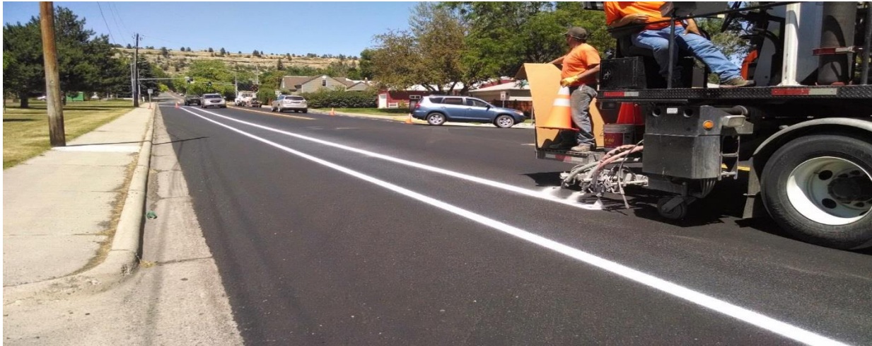
Image 2.3 Installation of bike lane as part of restriping project of 13 th Street West in July 2014
