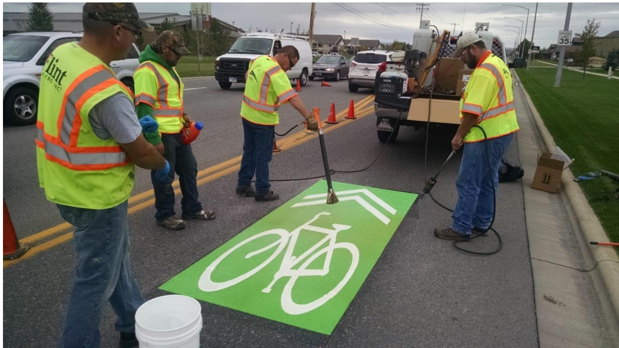
Figure 4.1 Shared lane panel install on 32 nd St. West at Central Ave
