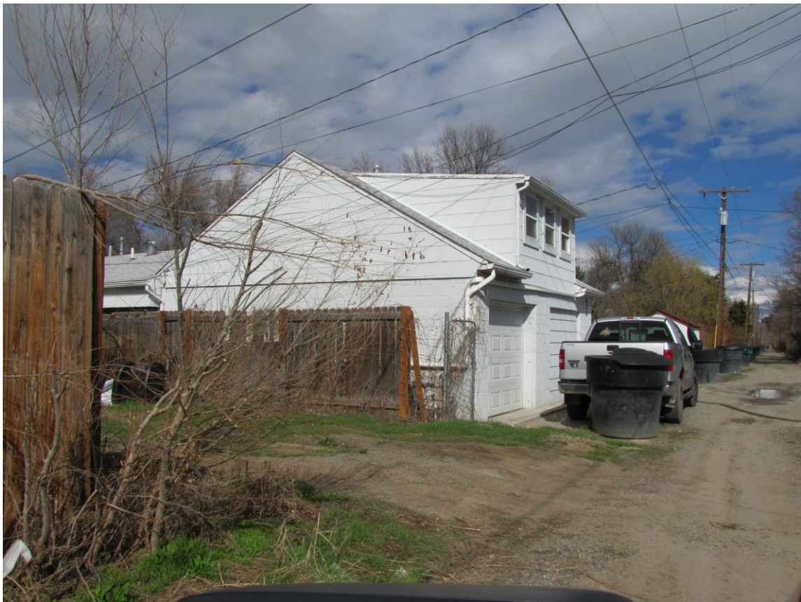
Property from the alley
