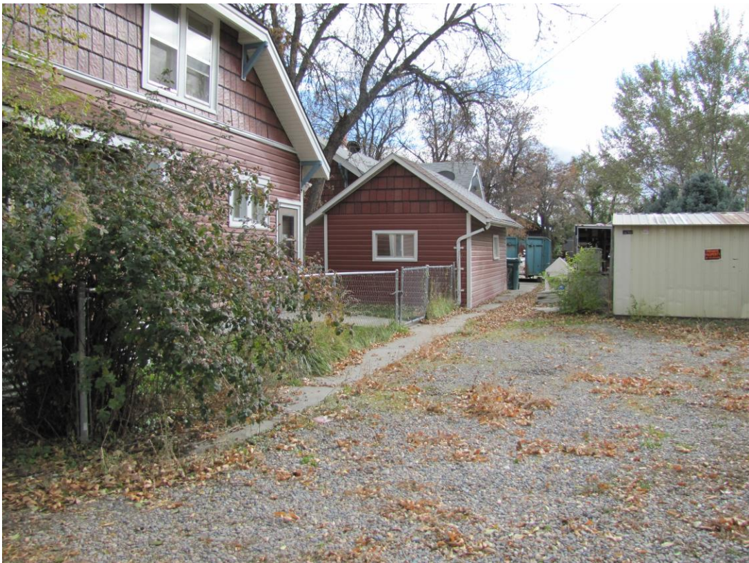
From the alley looking south
