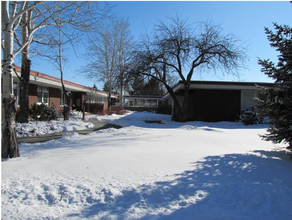
Structure to be renovated
