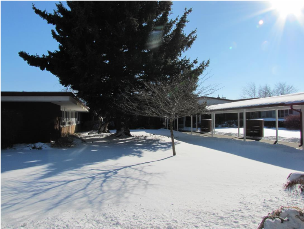
Structure to be removed
