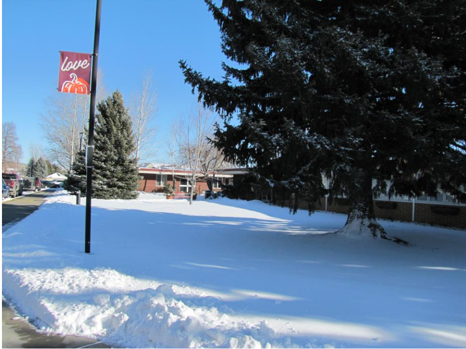
Structure to be renovated
