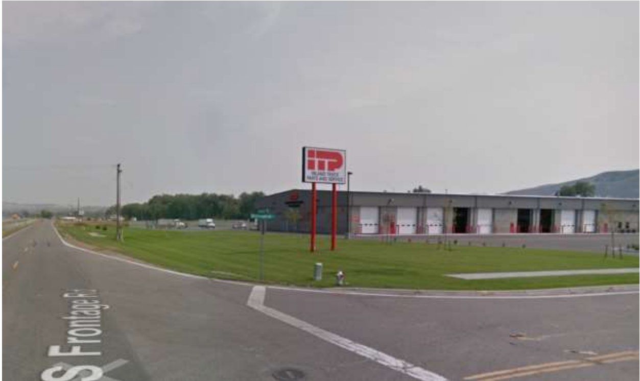
1011 Intermountain Street (S Frontage Road) West of subject property – No permit of record
