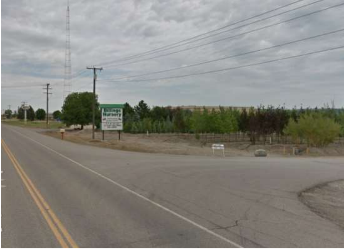
7900 S Frontage Road – A-1 zone ~ 128 sf
