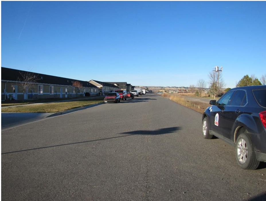
View north along S 44 th St West
