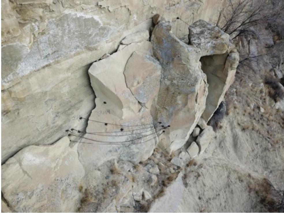
Photo looking west showing tensioned cable and bent plate.
