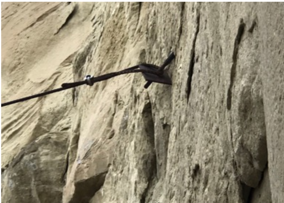
Photo looking west showing tensioned cable and bent plate.
