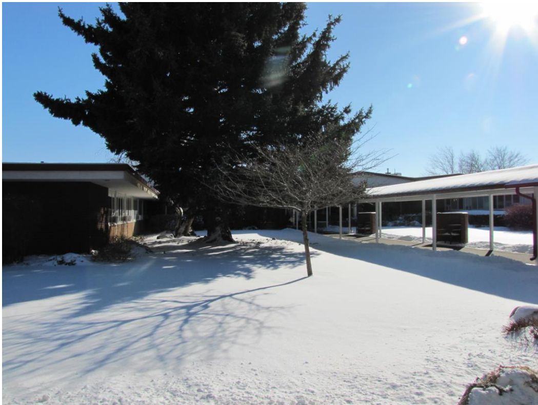
Structure to be removed
