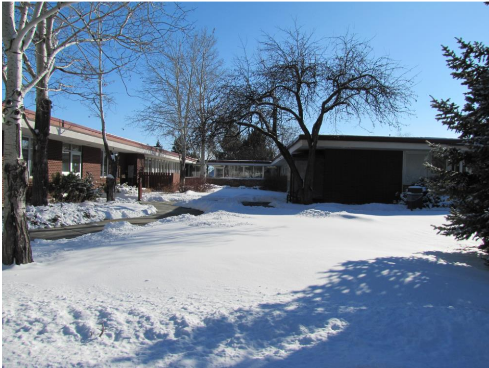
Structure to be renovated
