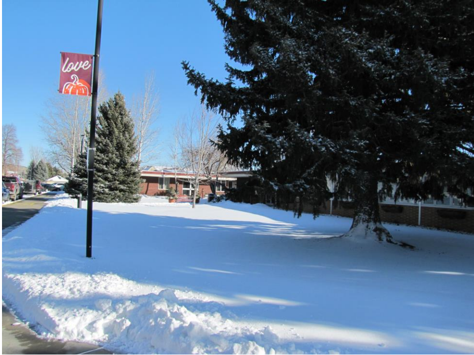
Structure to be renovated
