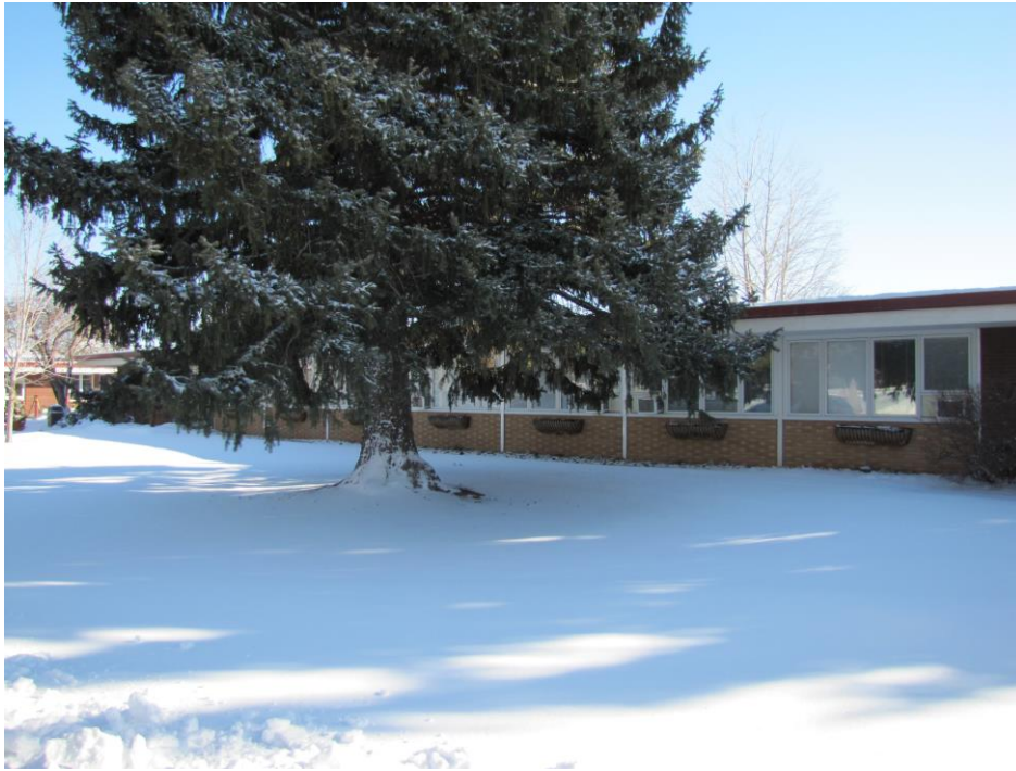
Structure to be renovated
