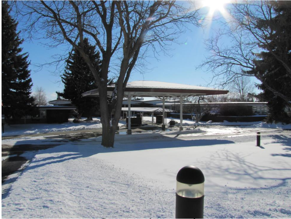
Structure to be removed
