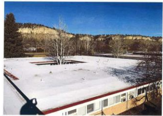
Exterior view Wing 2 looking north to Rimrock Road
