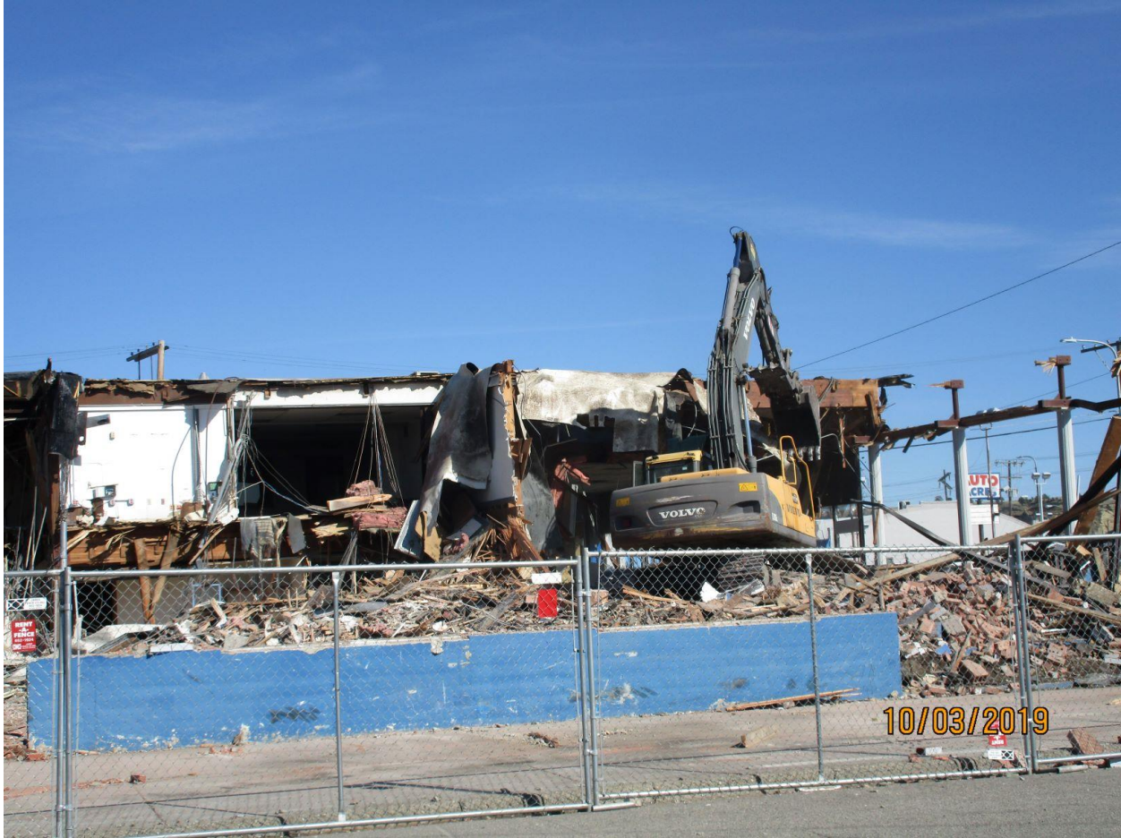
Property demolition underway – Looking southwest across property.
