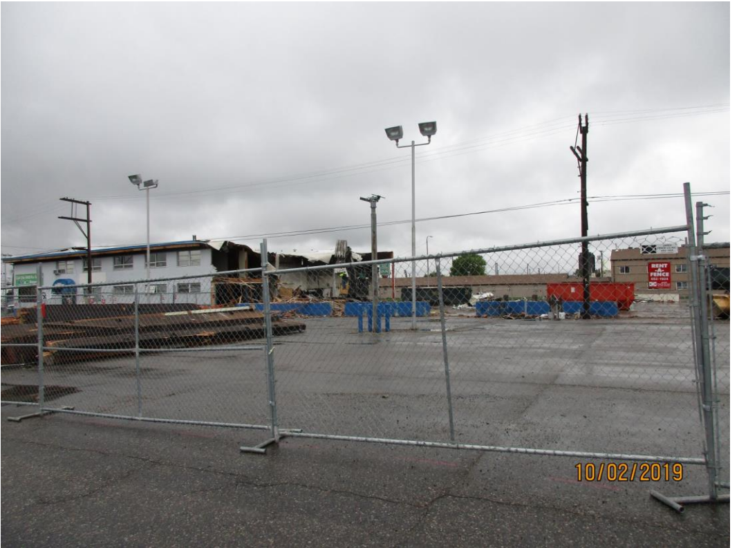
Property demolition underway – Looking west across property.
