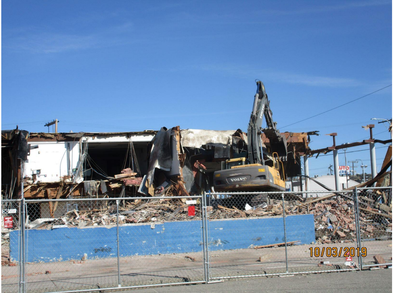
Property demolition underway – Looking southwest across property.
