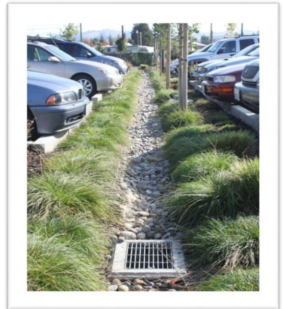
Fig. 27-1106.B Left: Landscape islands with storm water infiltration; Fig. 27-1106.C Right: Landscape divider with bio-swale
