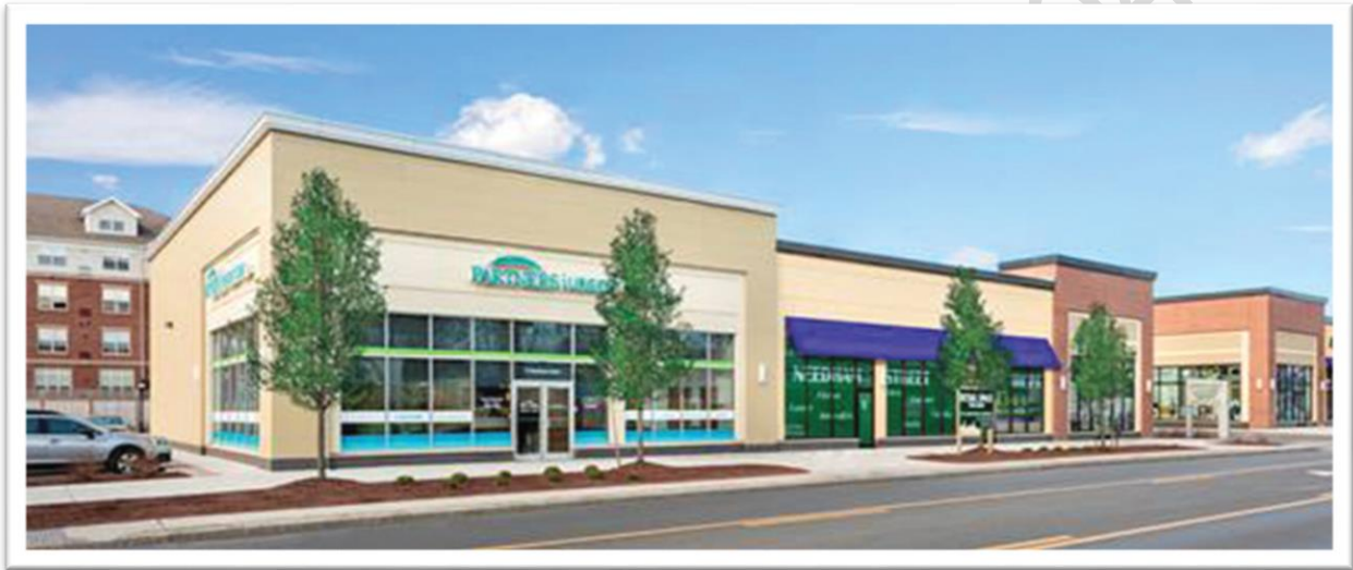
Fig. 27-1104.A: Sample illustration of new street trees installed on a commercial site.
