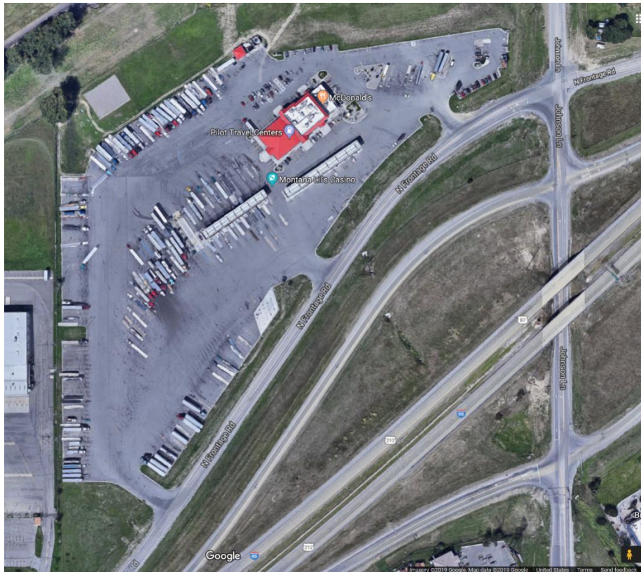
Pilot Truck Stop – Lockwood – built 2008 Controlled Industrial
