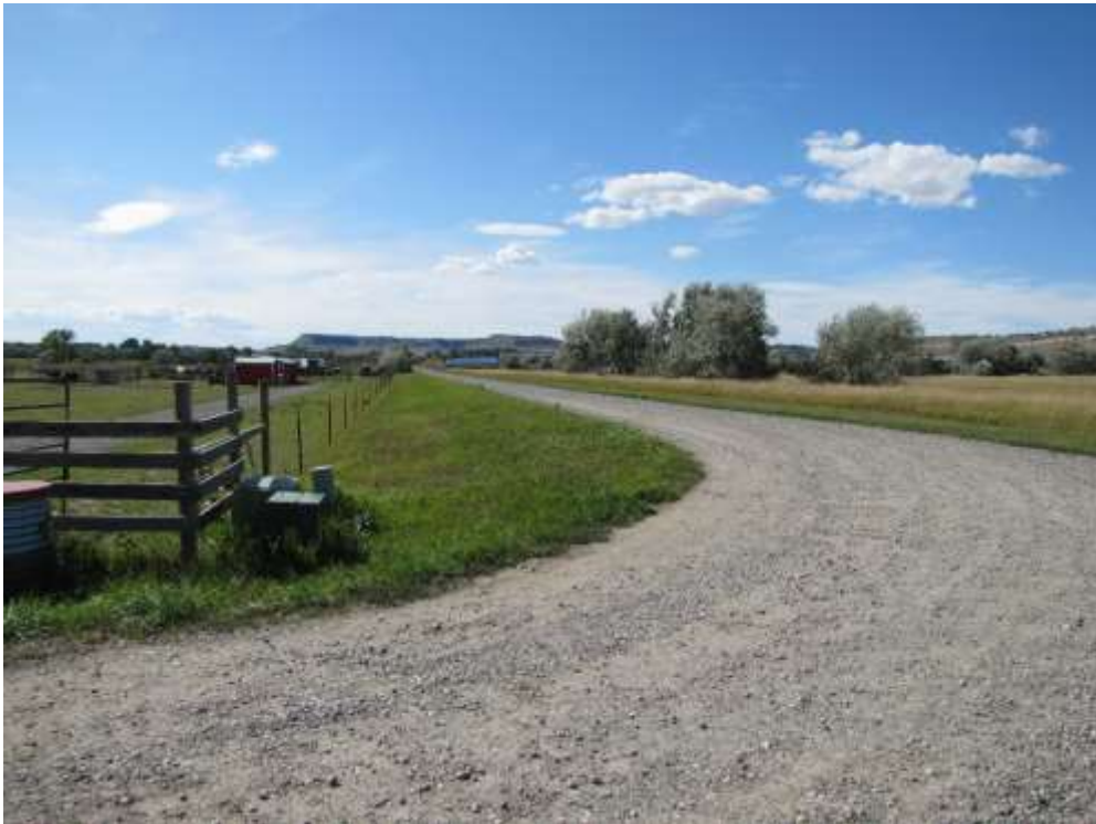
View west along Colton Blvd at intersection
