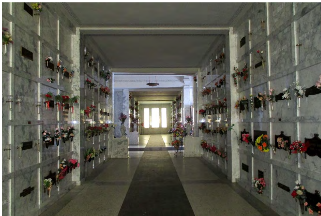
Photo 10 of 12: South corridor facing chapel and north corridor, 2019; view to north
