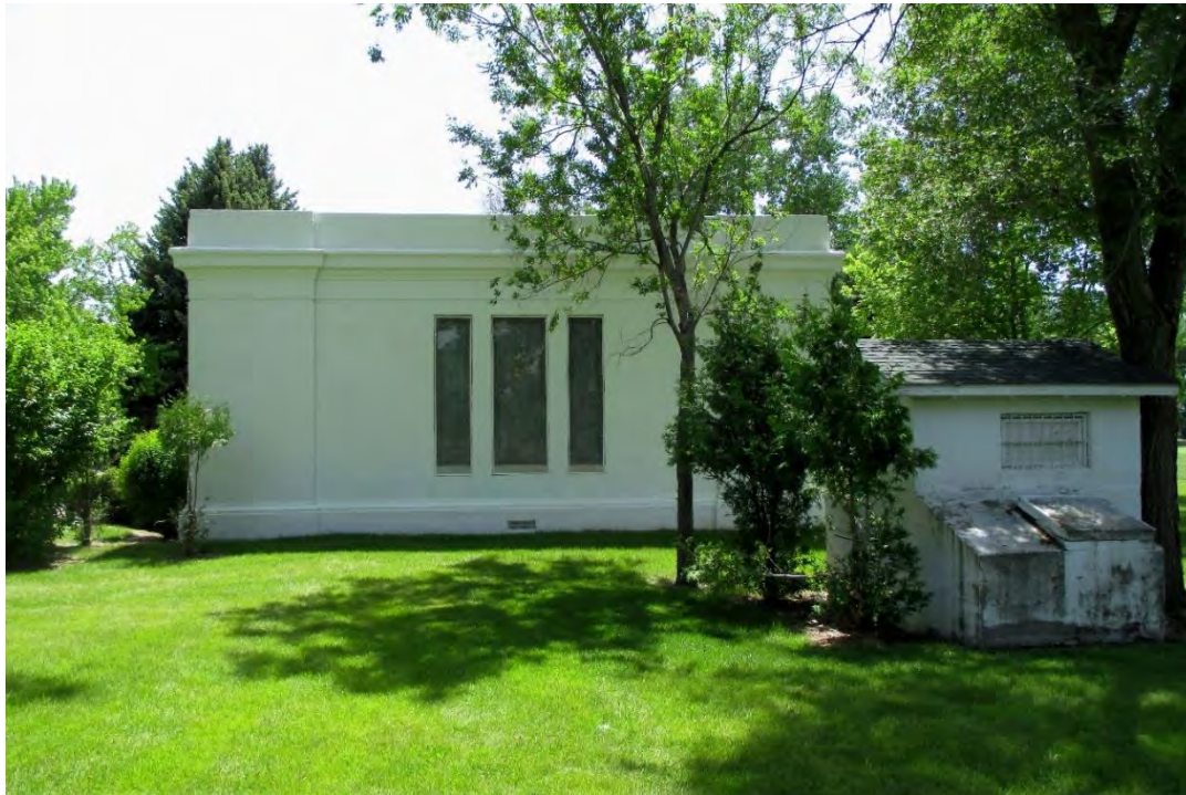
Photo 5 of 12: North elevation with pump house in the foreground, 2019; view to south
