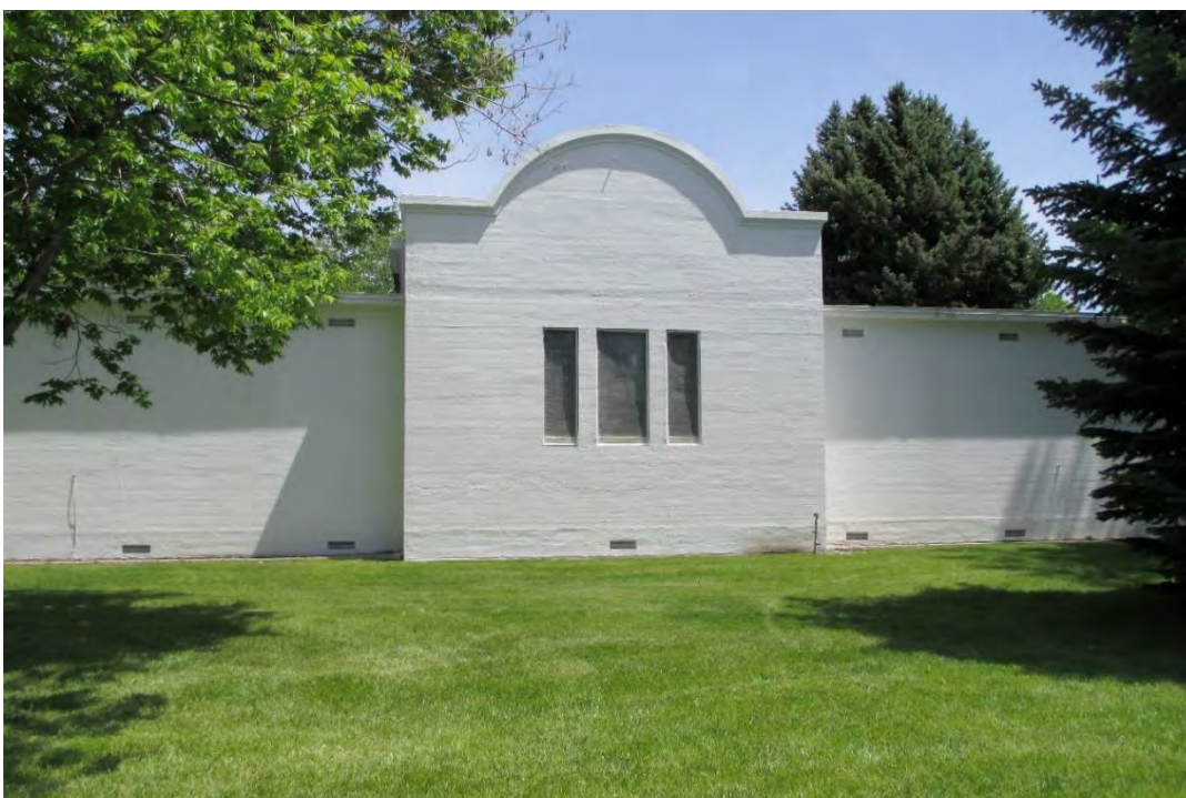
Photo 4 of 12: West elevation, 2019; view to east
