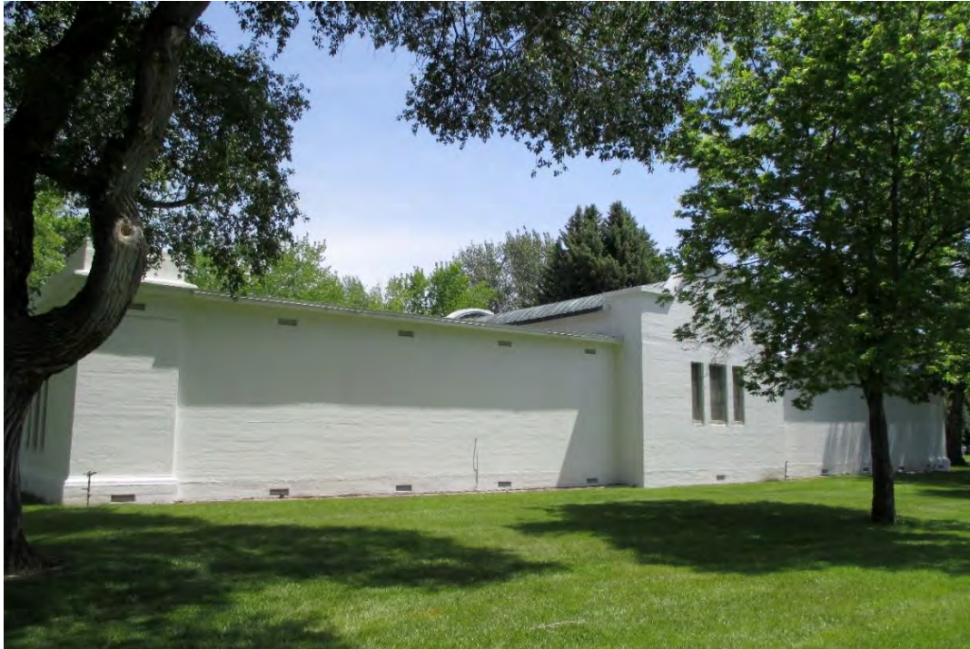
Photo 3 of 12: West elevation with view of barrel-vault roof, 2019; view to southeast
