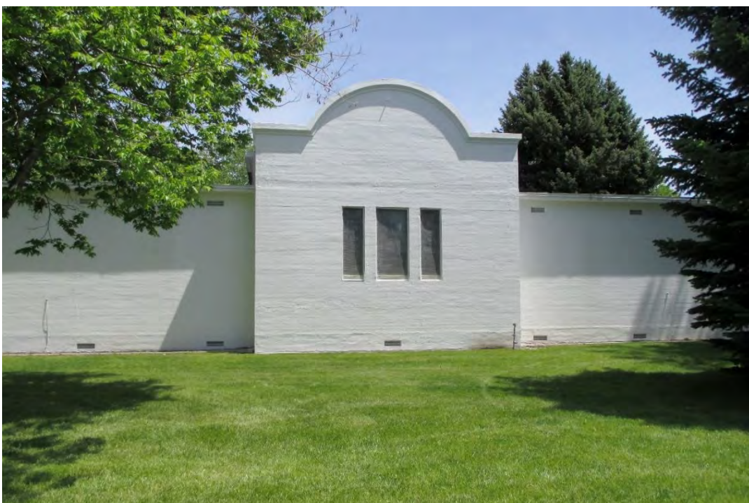
Photo 4 of 12: West elevation, 2019; view to east
