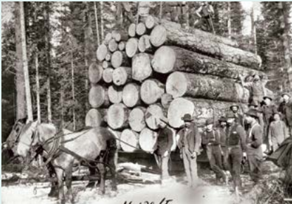
16,130 ft. of Logs, Hauled by Baker Brothers with a Single Team, March 17, 1900 MHS 949-126
