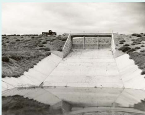
The overflow spillway at Anita Reservoir on the Huntley Project, built by Civilian Conservation Corps workers ca. 1934 MHS PAC 2003-47-135
